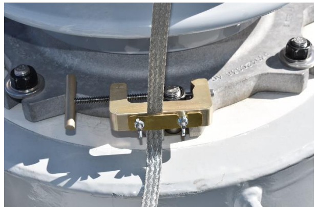
Earth connection to the ground clamp
